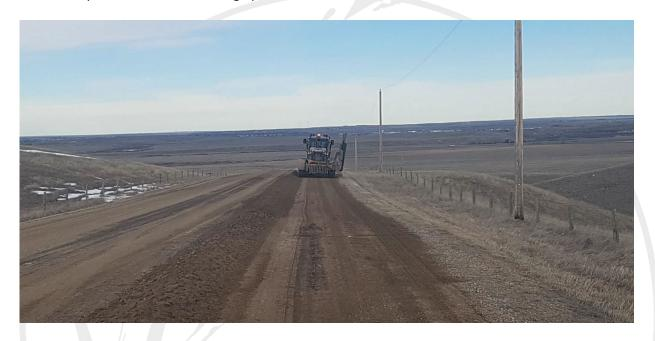
**Step 7:** At the end of the 4<sup>th</sup> cut, turn the grader around and straddle the windrow. This will be your 5<sup>th</sup> pass and you will begin to spread. As you are spreading, you are to keep the gravel approximately 1 metre away from the shoulder of the road.
