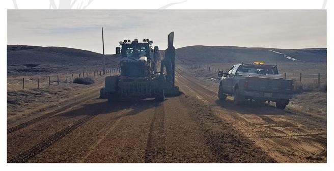
**Step 8:** At the end of the 5<sup>th</sup> pass turn the grader around and straddle the windrow. You now can pick up one of the signs and start your 6<sup>th</sup> pass which is the 2<sup>nd</sup> spreading pass. This is your final pass, so keep the gravel approximately 1 metre away from the other road shoulder. Once you have completed your final pass of spreading, you can pick up your other sign.
