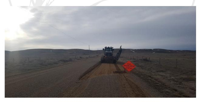
**Step 3:** At the end of the first cut pass, pull ahead approximately 20 metres and set up the second "Road Grading Ahead" sign.
