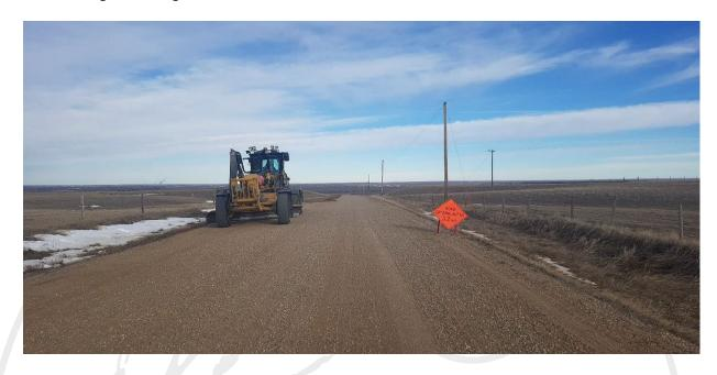
**Step 4:** Turn grader around and proceed with 2<sup>nd</sup> cut, with the grader straddling windrow. Roll windrow over and cut in the same direction as the first pass. Be sure to have enough down pressure to cut out any washboard and ruts. The advantage of carrying one windrow allows for the mixing of all bladed material throughout the entire road maintenance procedure. **At all times you will only have 1 windrow.**
