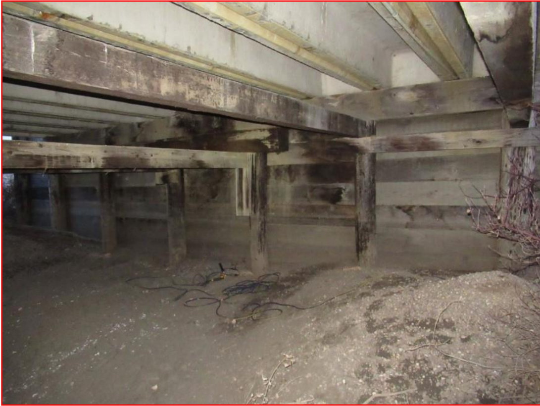
Photo 3: Looking at South Abatement (A1)
