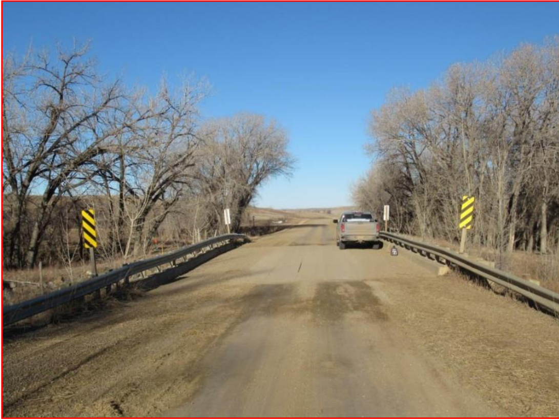
Photo 5: Alignment looking West
