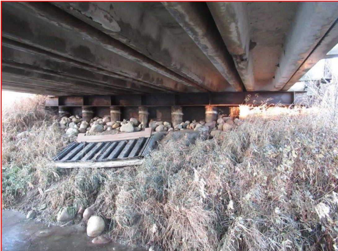
Photo 2: North Abutment (A2)
