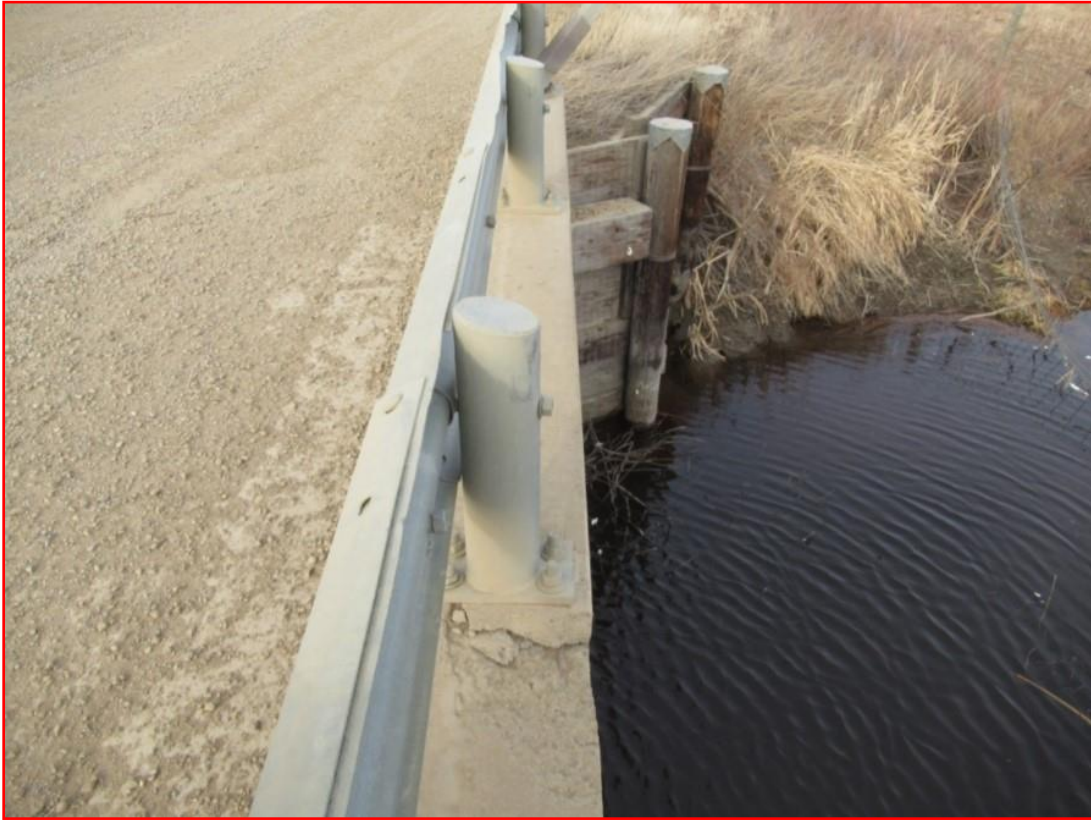
Photo 1: Looking at Curb Fascia (Concrete Repairs)
