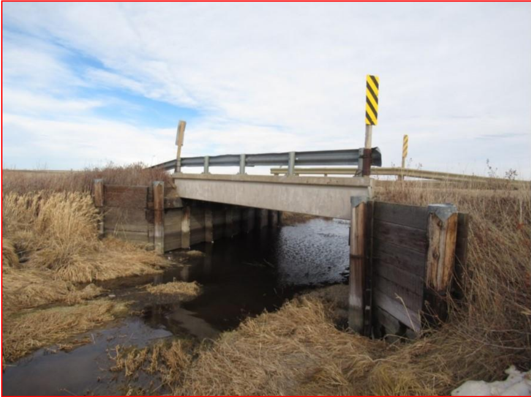
Photo 3: Looking at Abutment #2
