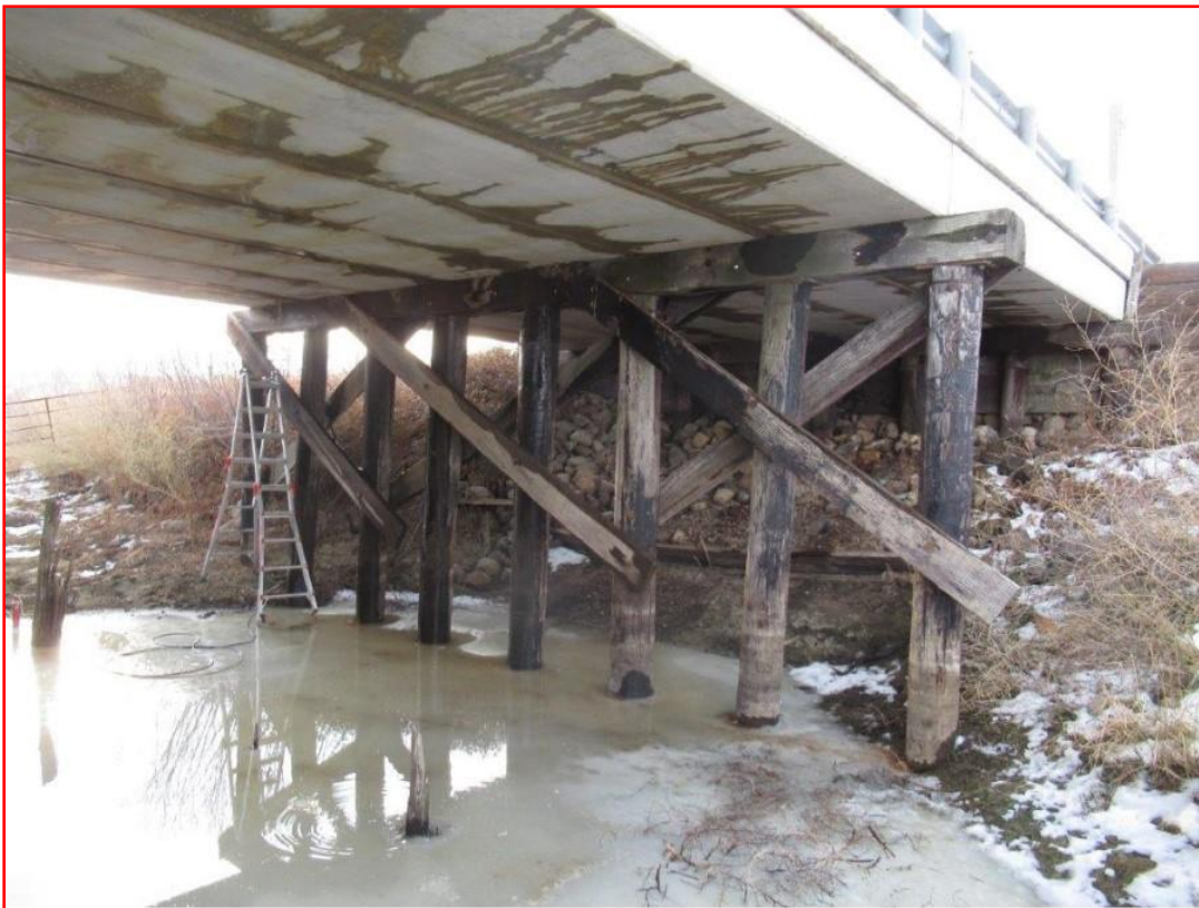
Photo 4: Looking at Pier #1
