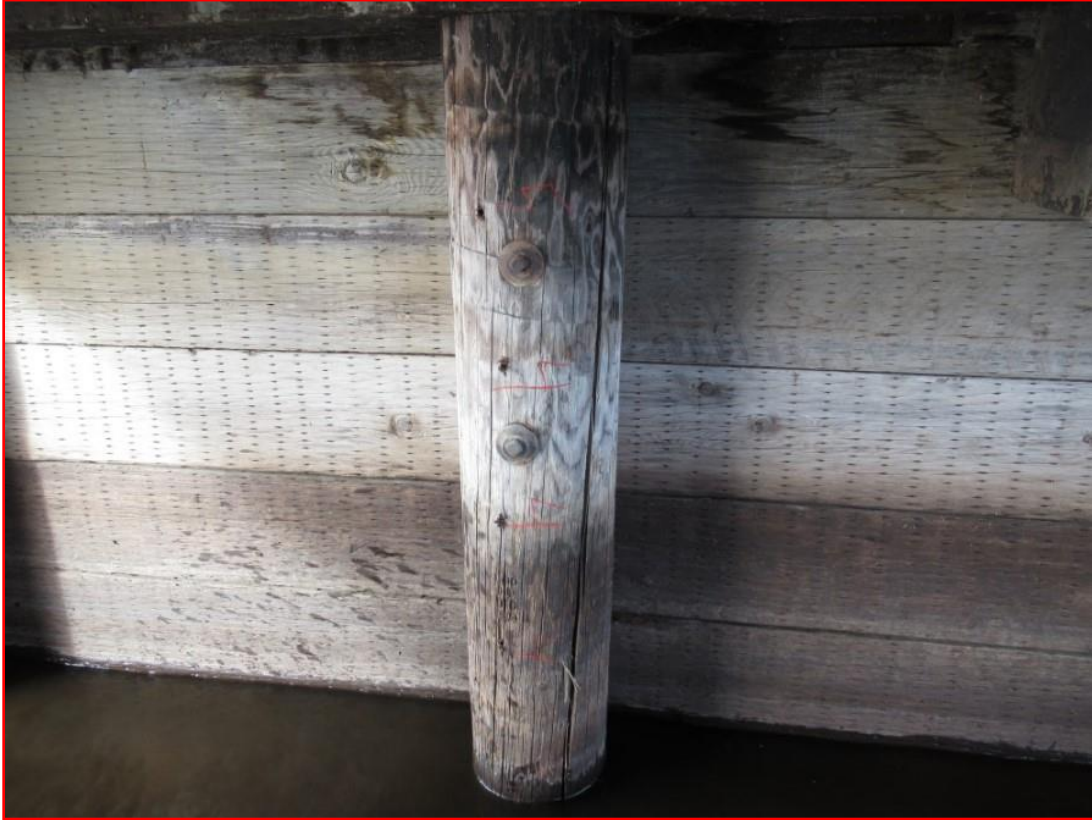
Photo 5: A2-P2 Install H-Pile Stub
