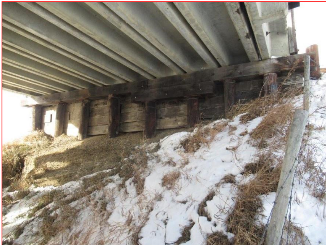
Photo 4: Looking at Abutment #2
