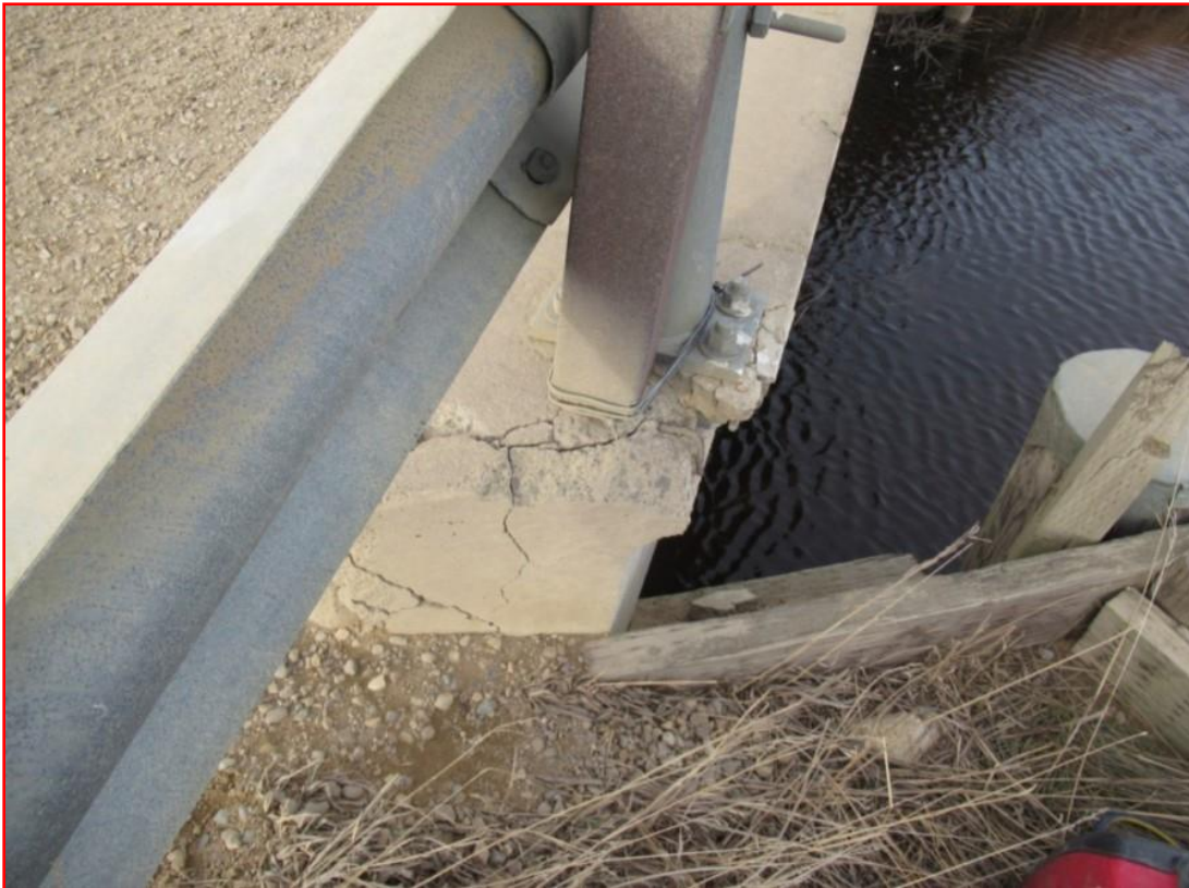
Photo 2: Looking at Curb Fascia (Concrete Repairs)
