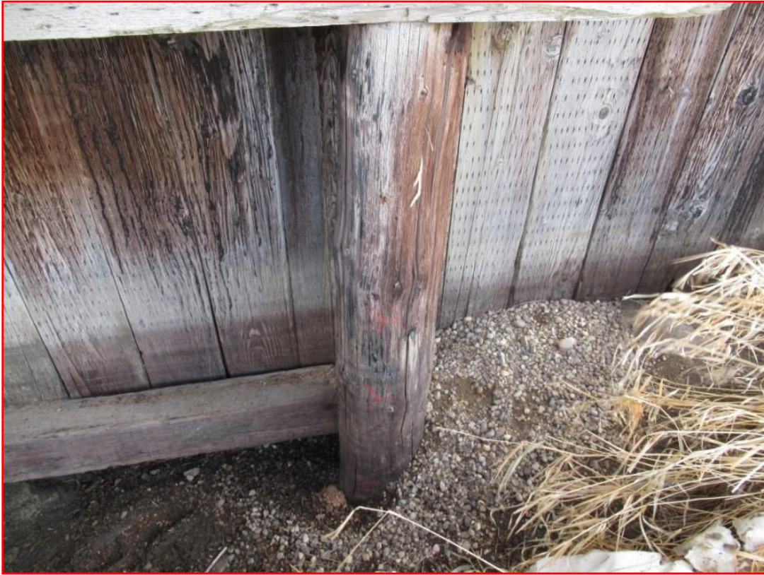
Photo 3: A1-P1 Install H-Pile Stub
