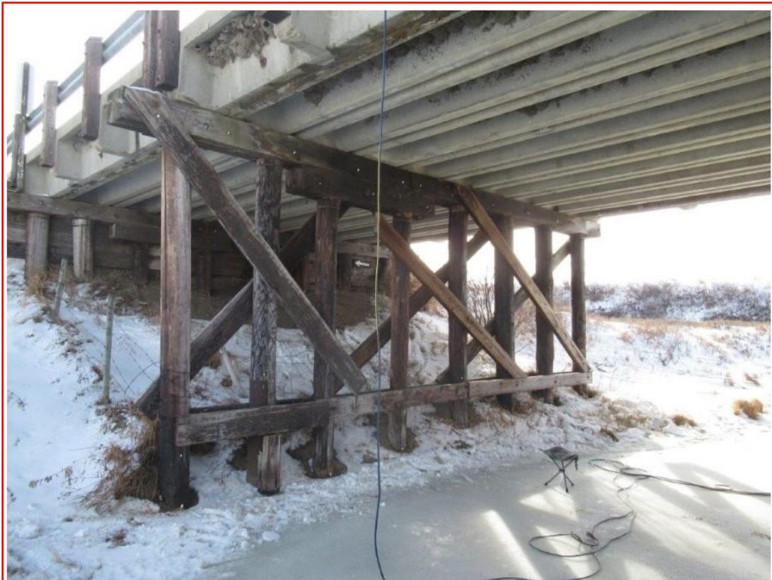
Photo 2: Looking at Pier #1
