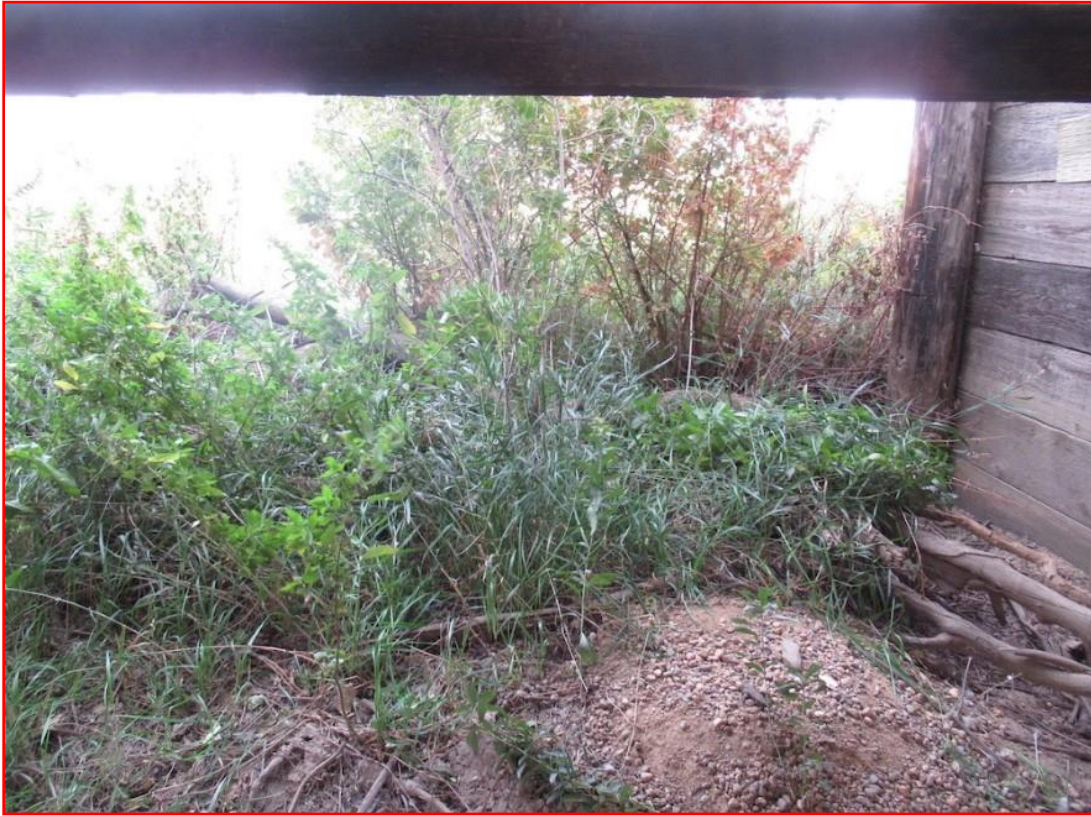
Photo 1: Drift Under Bridge
