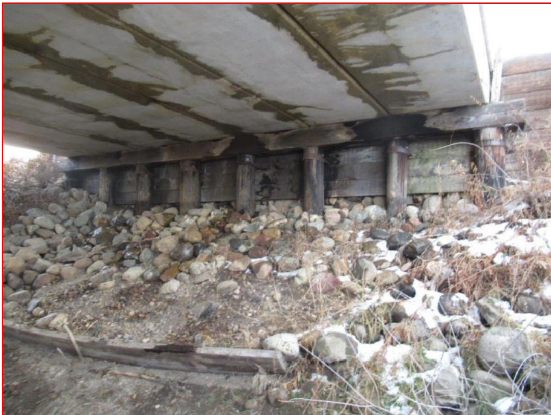
Photo 2: Looking at Abutment #1
