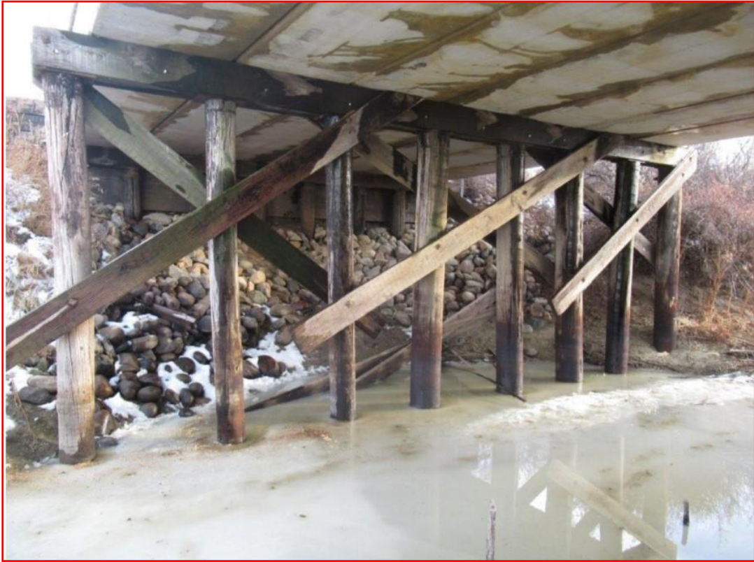
Photo 5: Looking at Pier #2
