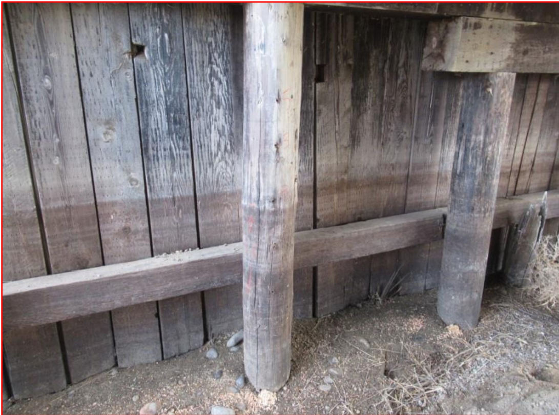
Photo 2: A1-P7 Install H-Pile Stub
