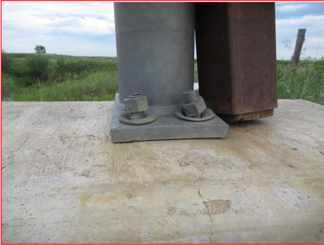
Photo 1: View of Anchor Bolts
