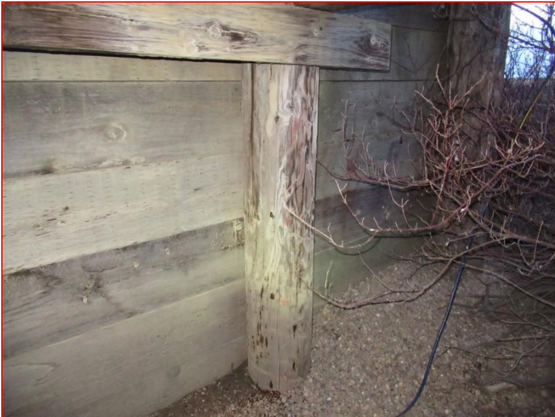
Photo 2: A1-P1 Install H-Pile Stub
