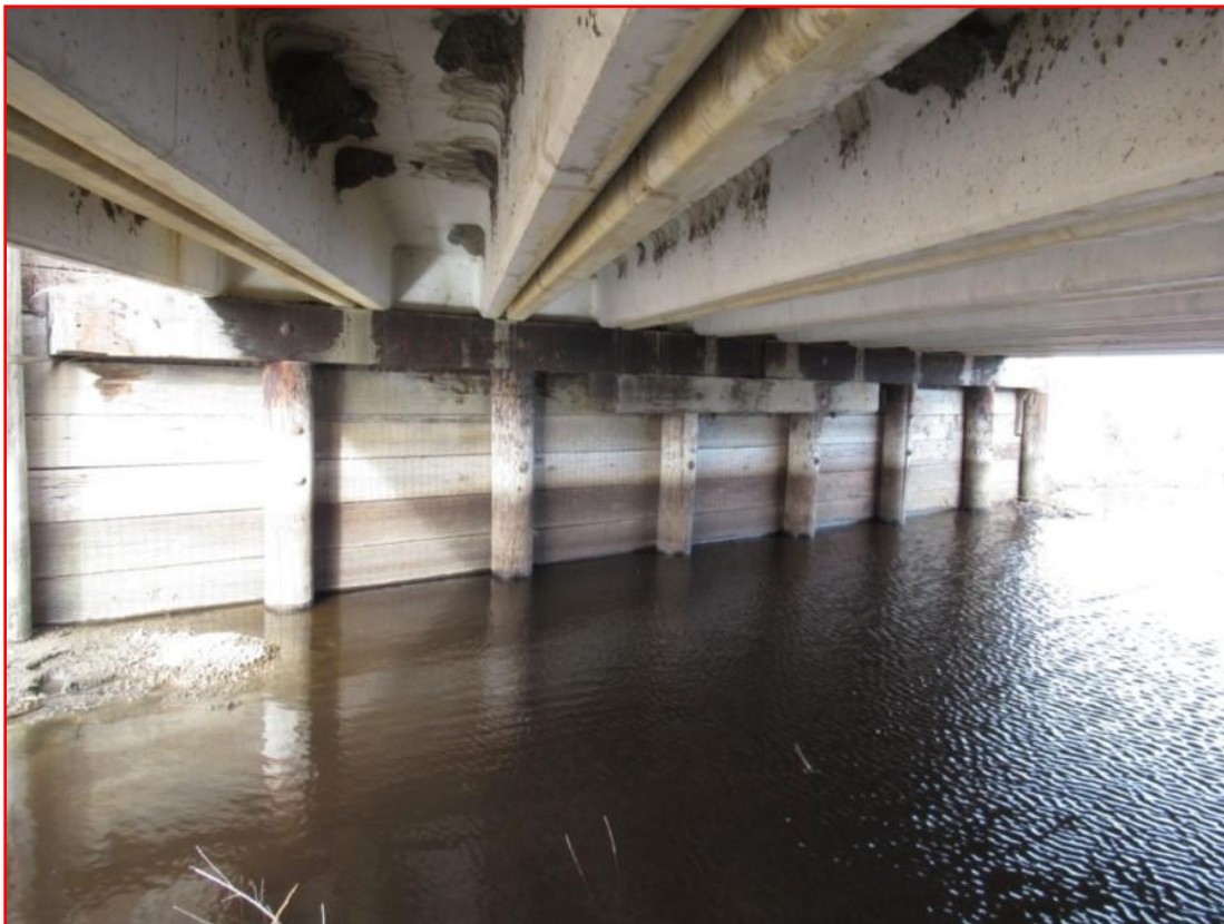
Photo 4: Looking at Abutment #2
