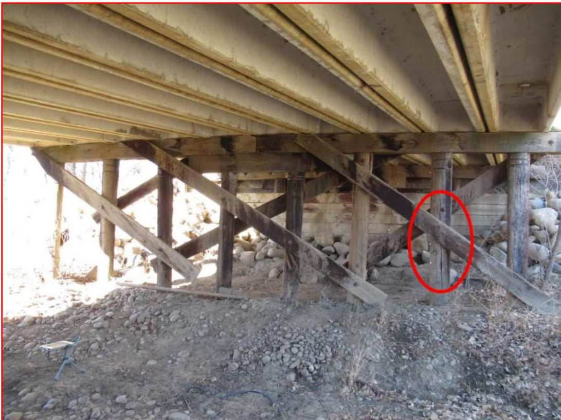
Photo 2: Looking at Pier #1
