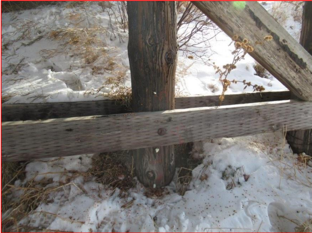
Photo 1: P1-P2 Install H-Pile Stub
