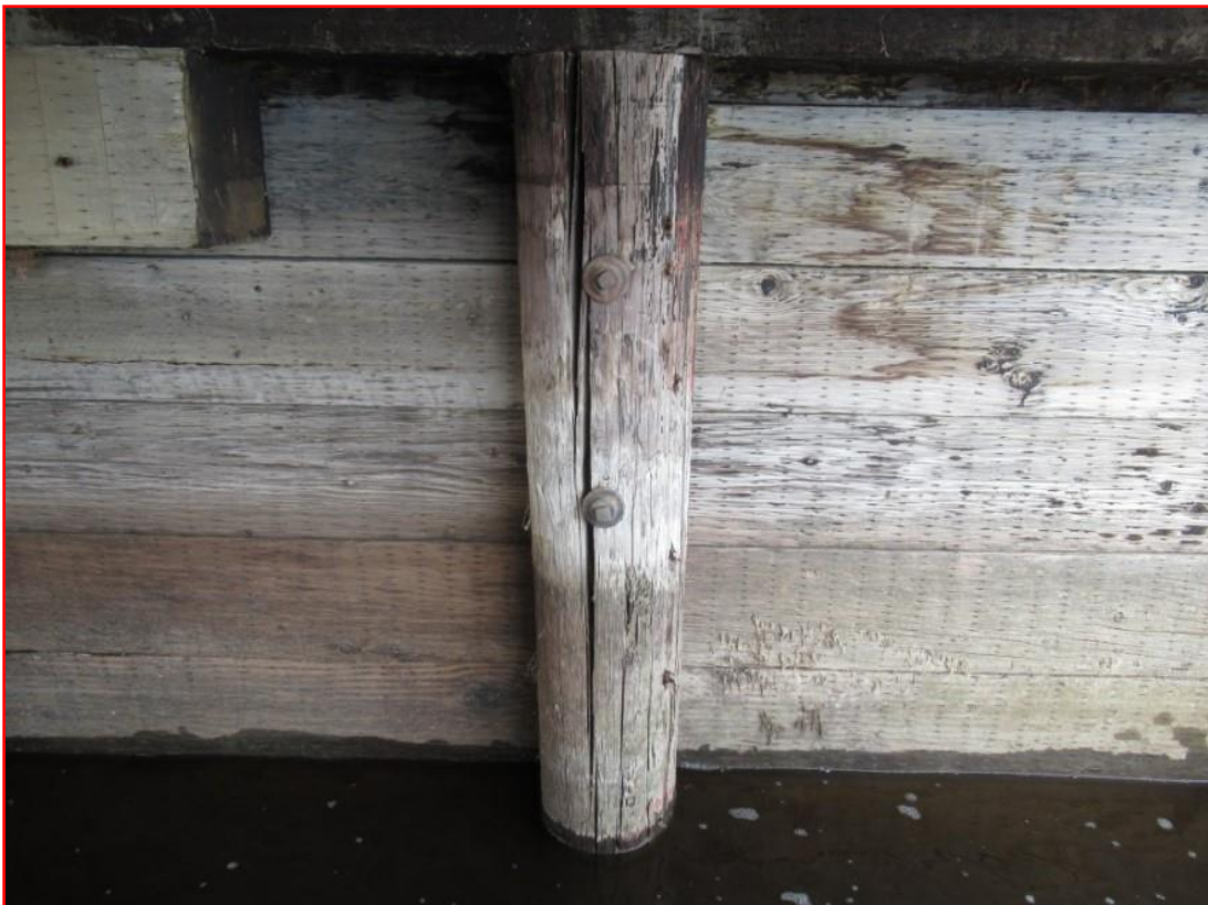
Photo 6: A2-P5 Install H-Pile Stub
