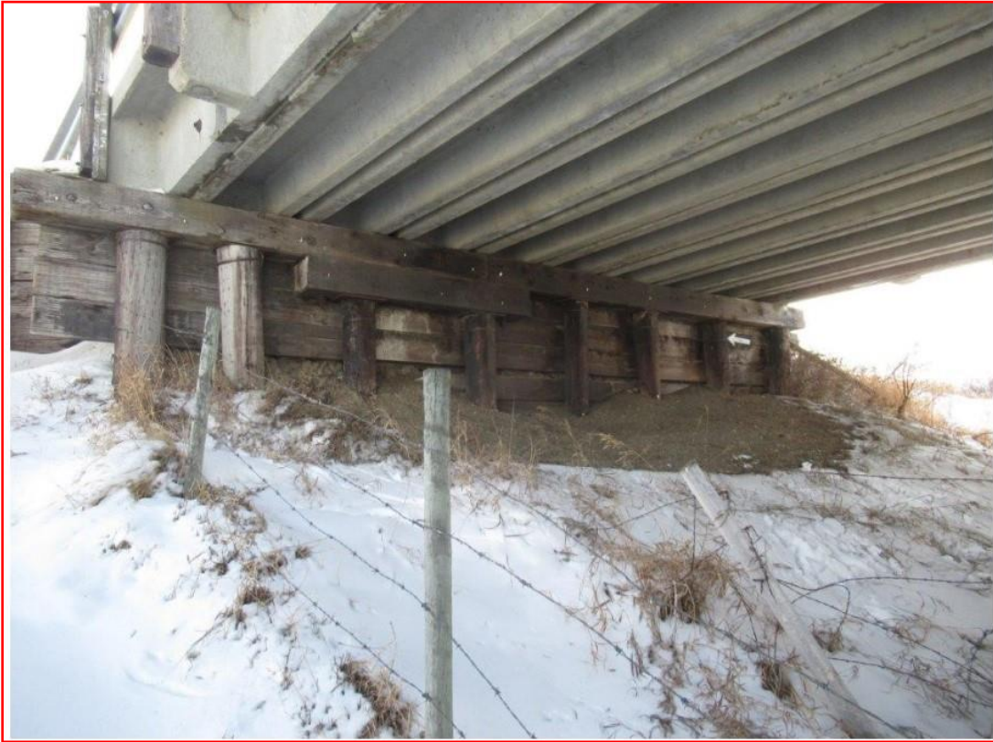
Photo 3: Looking at Abutment #1
