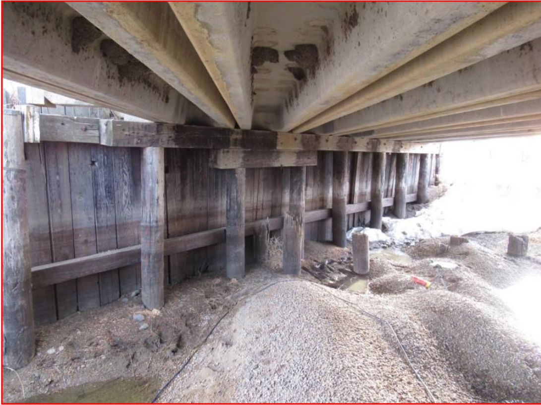
Photo 1: Looking at Abutment #1
