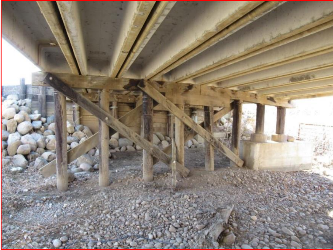
Photo 3: Looking at Pier #2
