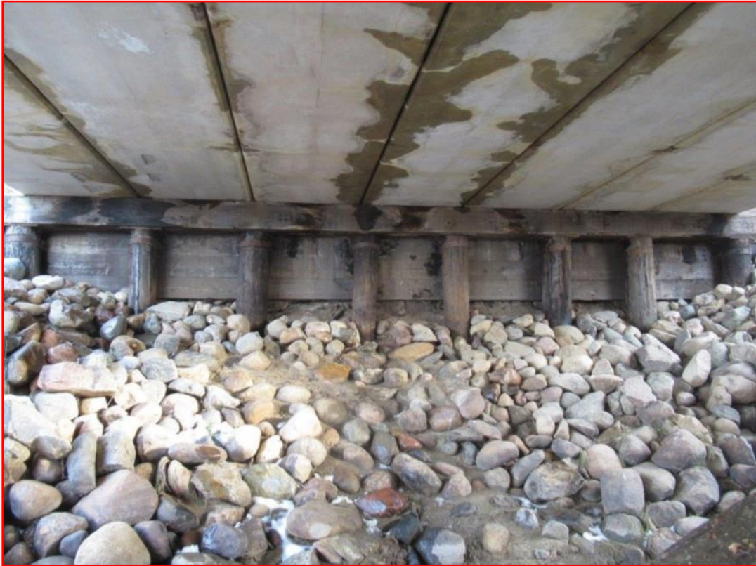
Photo 3: Looking at Abutment #2
