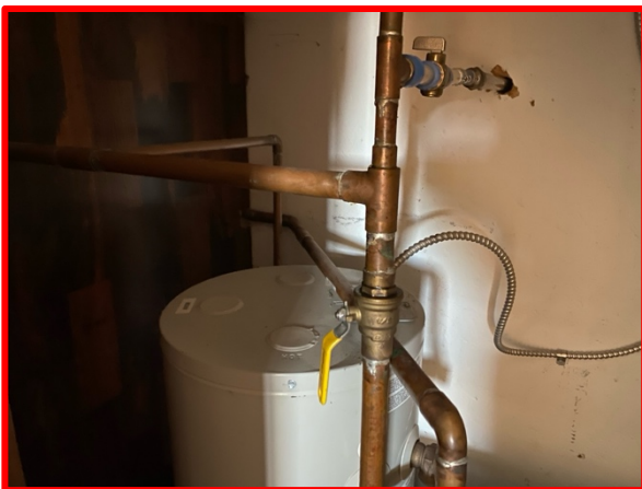
Water Lines Soldering
