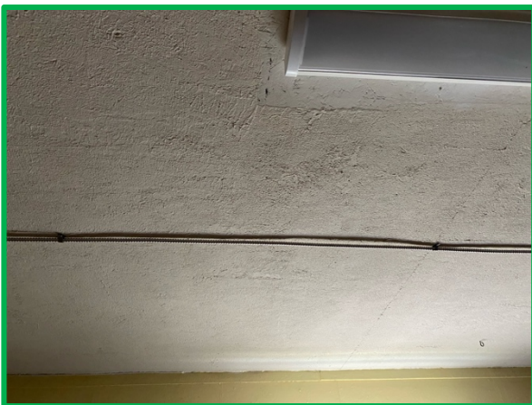
5-1 – NW Room; Ceiling / Texture
