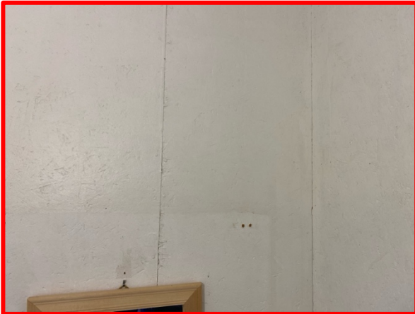
L3 – Bathroom Walls & Ceiling / White Paint
