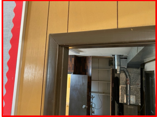
L2 – Interior Doors & Jambs / Brown Paint
