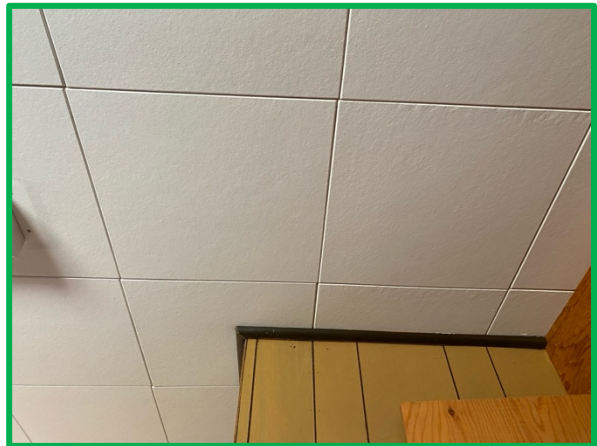
4-1 – SW Room; Ceiling / 12x12 Tile
