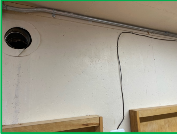
L1 – Interior Walls & Ceiling / Beige Paint
